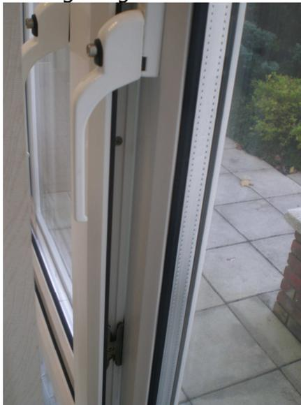
This allows the flow of air in and out, but also means that the window is locked from the outside.
