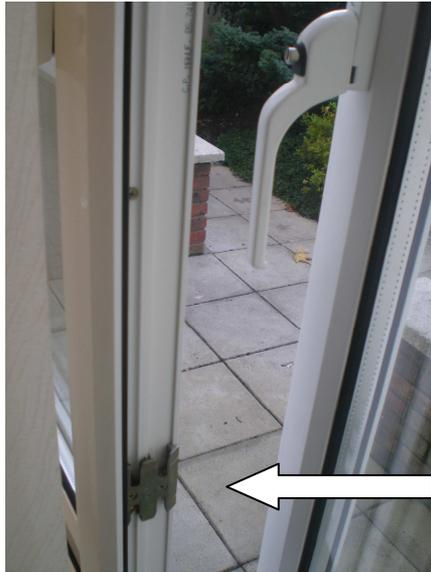
At the bottom of the image above you can see the double latch on the frame of the window. When you have your window fully closed the lock sits in the first latch, on the left in this photo.
